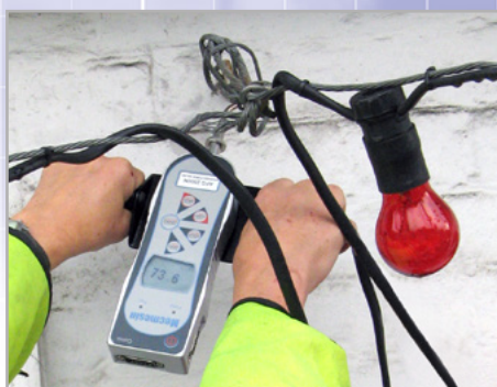
Pull test on anchorage points
